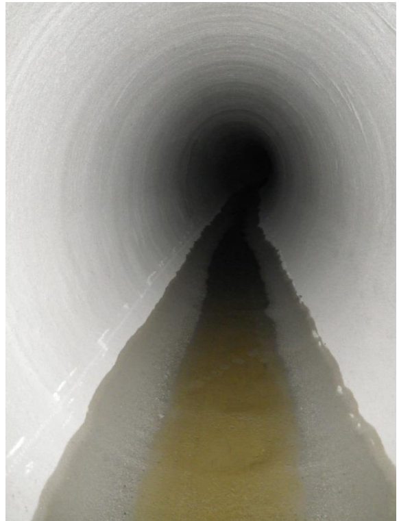
After cleaning & rehab
