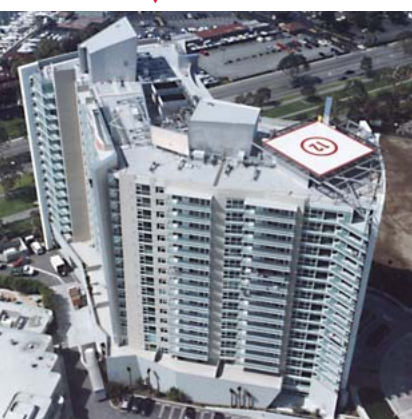
This high-rise luxury condominium tower on the beach at Marina Del Rey, California is protected by a complete Siplast System of torch grade Paradiene and Siplast Lightweight Insulating Concrete.
