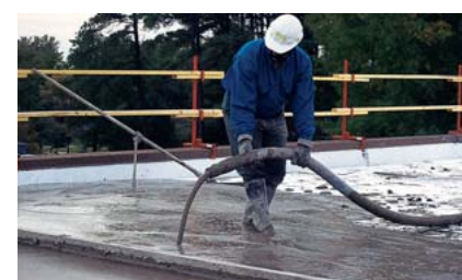
▲ A top layer of insulating concrete is placed over the Insulperm, filling the holes in the Insulperm and locking it into the system without the use of fasteners.
