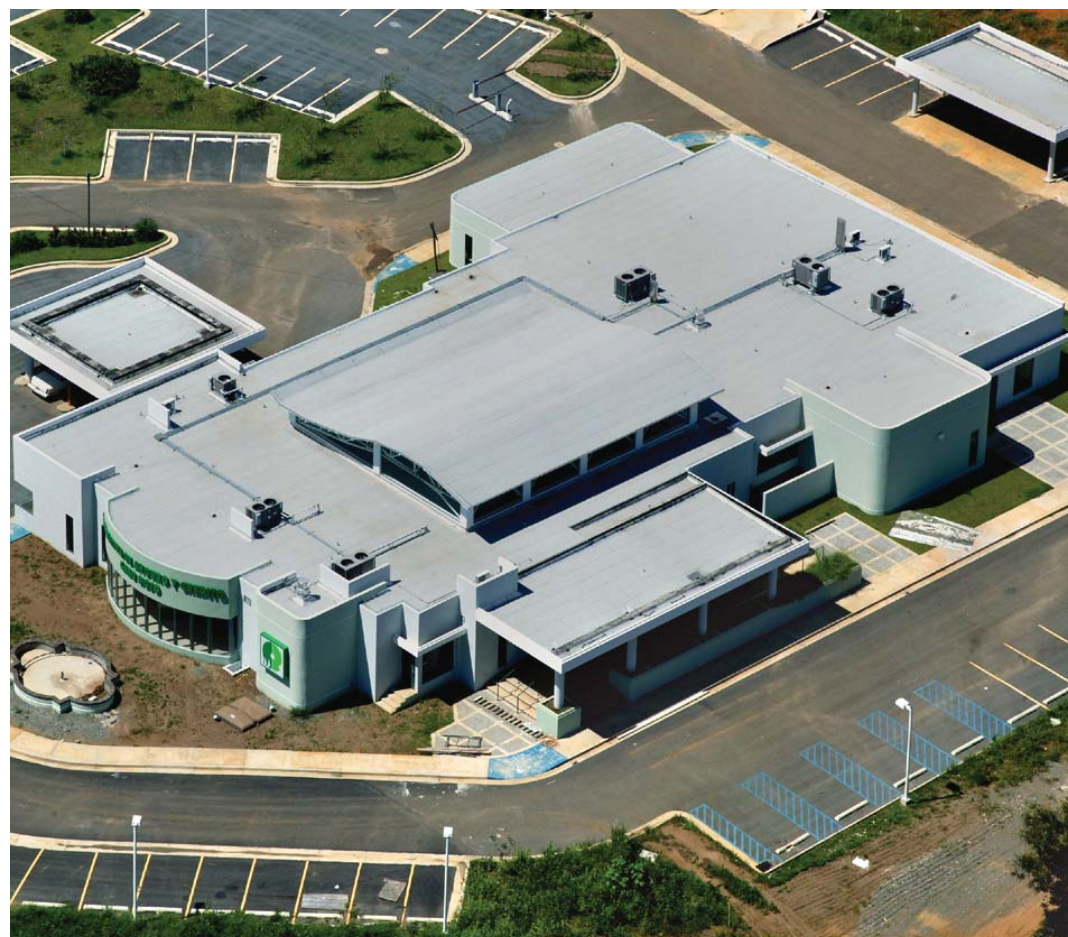
▲ The Insulcel-RT Lightweight Insulating Concrete System and a Paradiene 20 TS/ 30 TG Roof Membrane System were chosen for this bank in Puerto Rico.
