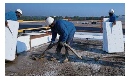
▲ Decreasing thicknesses of Insulperm Insulation Board form the slope-to-drain contour of the finished system.
