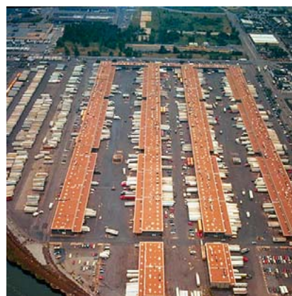
▲ Siplast Lightweight Insulating Concrete and over 7,000 squares of torch grade Paradiene work as a complete system to protect this fruit and vegetable market in the Bronx.
