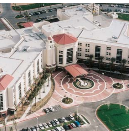
▲ A Siplast Lightweight Insulating Concrete System and Paradiene 20/30 FR Roof System were installed on this Nevada hospital.
