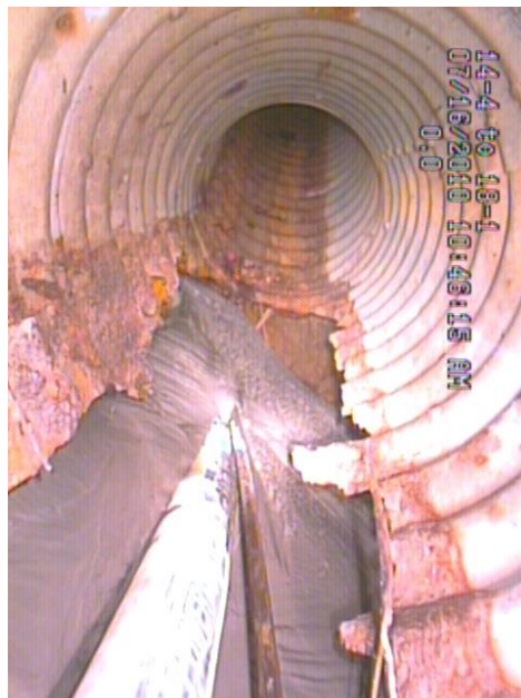
Self-leveling grout pumped into invert of 12" CMP
