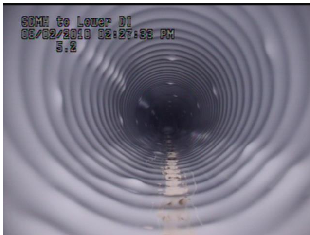
PVC fold and form installation complete in 12" CMP
