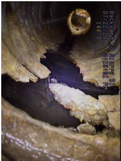
Deteriorated invert in 12" CMP
