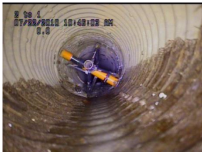
Deteriorated invert in 12" CMP
