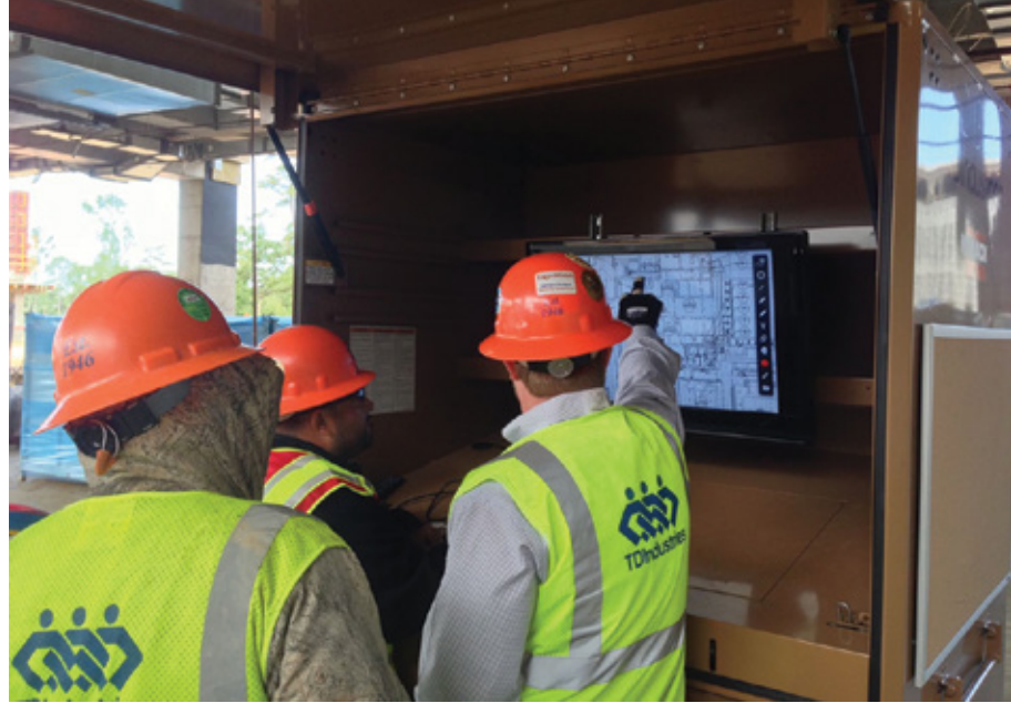
TDIndustries Field Personnel View Construction Drawings in Onsite Job Box from iPads.
