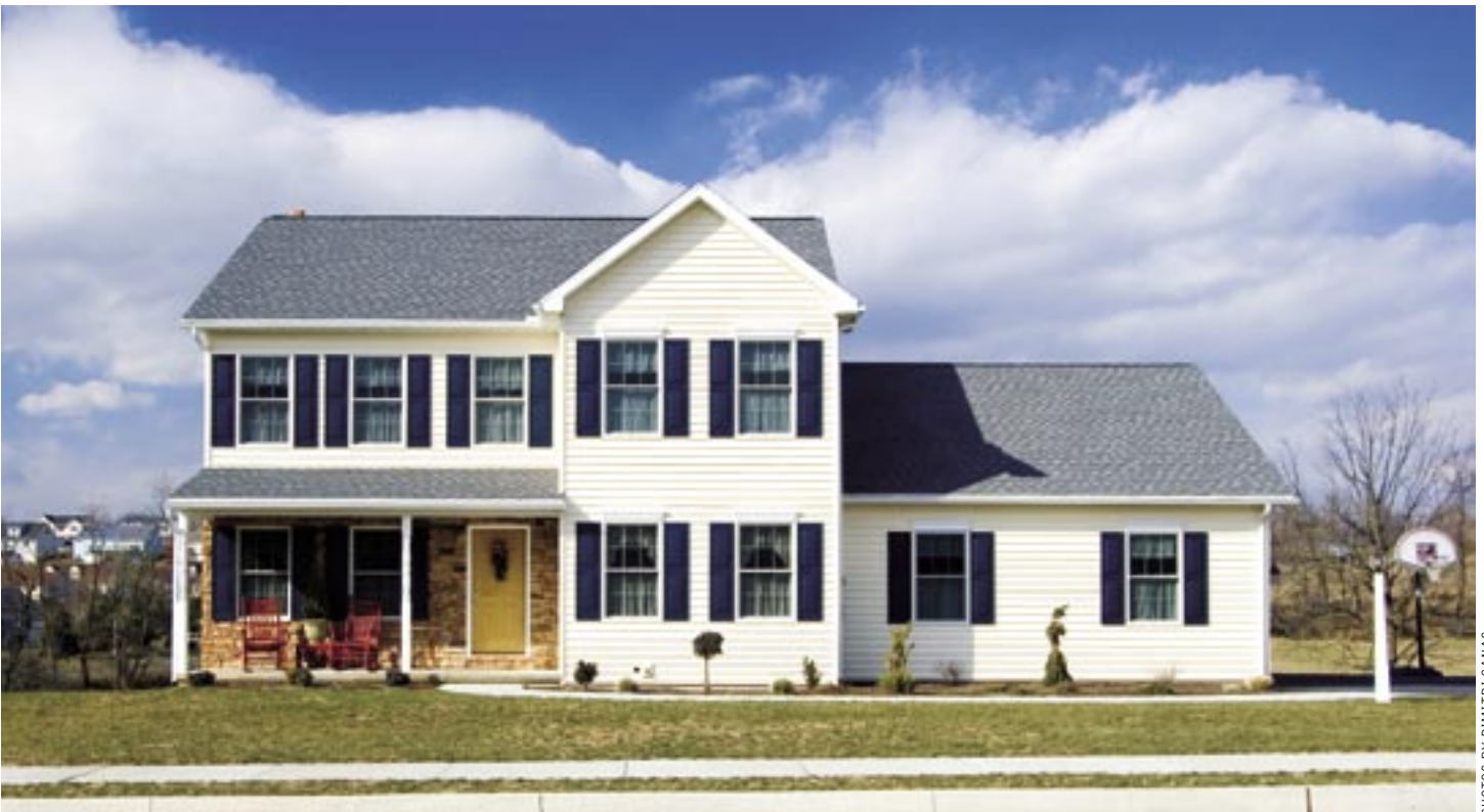
Another Landis Builders, Inc. custom home in Chestnut Ridge has a side-loading garage. This attractive home has four bedrooms, two-and-a-half baths and is 2,100 square feet.
