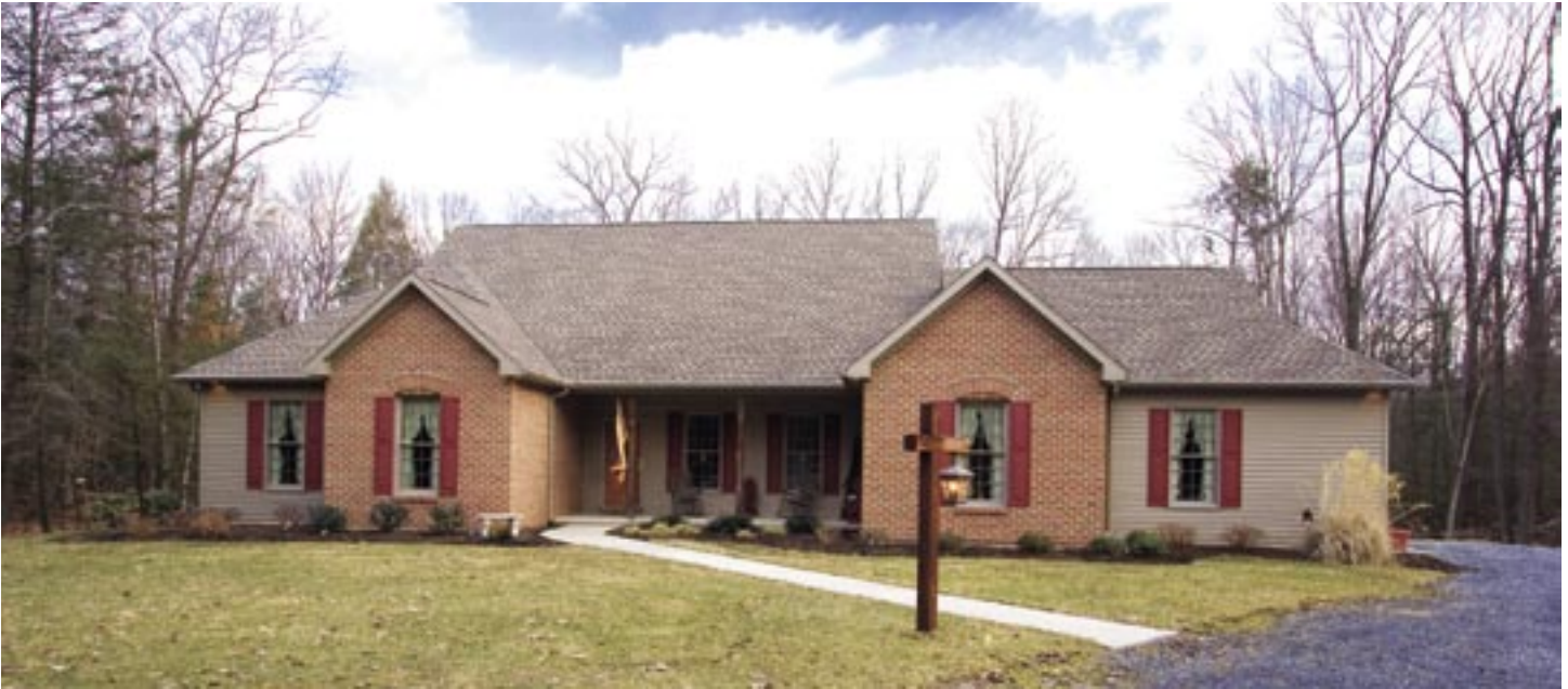
This custom home by Landis Builders, Inc., is about 2,000 square feet. Brick and siding, with a side-loading garage create an attractive exterior in this country, woody setting near Jonestown. The home has three bedrooms, and two-and-a-half baths and is designed for first-floor living.
