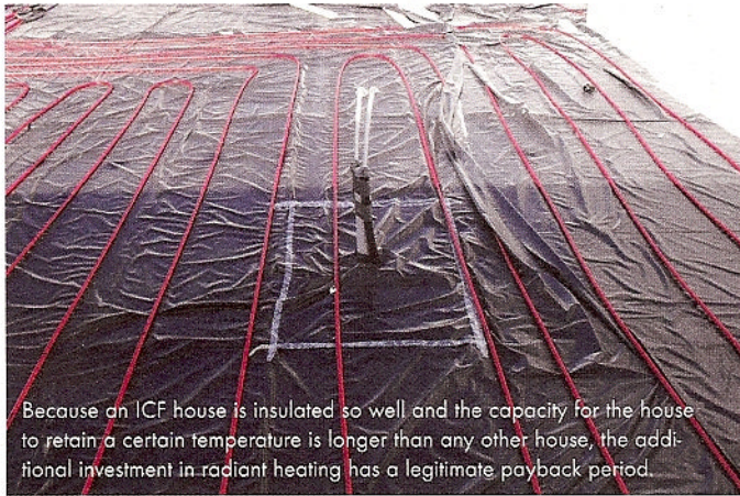
RadiantPEX+ is manufactured to meet the American Standard Testing Method for cross-linked polyethylene tubing (ASTM F 876-09), and all sizes are made to the Standard Dimension Ratio for plastic pipes.
