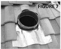
**FLAT ROOF INSTRUCTIONS:** When the hole is cut, apply two concentric beads of supplied roof caulking to underside of flashing. Center flashing with hole and secure to roof with (8) #8 x 2" self-tapping stainless steel or corrosion resistant screws (*supplied*). Apply a 4" reinforcement fabric and high quality roof mastic (*not supplied*) around perimeter of flashing to double seal any potential water leaks. Finish installation by following **STEPS 2** and **3** of Shingle Roof instructions.
