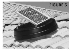
**TILE ROOF INSTRUCTIONS:** Remove several tiles and follow instructions same as on **STEP 1** for Shingle Roof installation, then unroll/unfold aluminum skirt with EPDM material and install over flashing (**Figure 7**). Cut and replace tiles according to local roofing codes. Use supplied roof caulk to seal where needed and follow **STEPS 2** and **3** of Shingle Roof instructions to complete installation.
