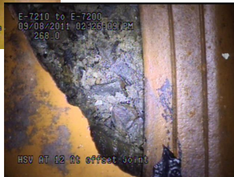
Pipe piece missing at 12 o'clock
