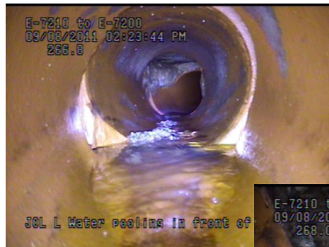
Pipe piece missing at 12 o'clock
