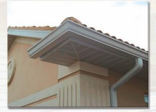
The purpose of guttering systems is to collect water (rain) from the roofing area and disperse the water away from your home. Properly configured gutter and downspouts are very essential. A faulty guttering system can contribute to damage to soffit & fascia, shingles, building foundations, driveways, walkways and landscaping.
