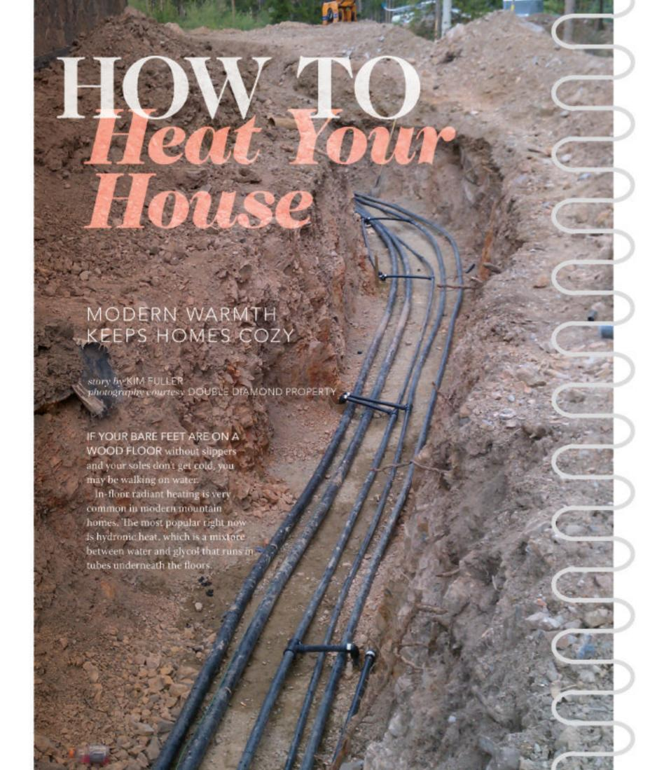
PREVIOUS PAGE: This photo features supply runs from the geothermal wells running back to the house. These use ground heat to help supplement the use of bollers.
