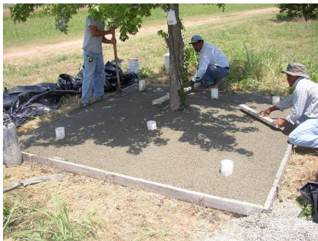
Figure 4. Finishing concrete and installing access ports.
