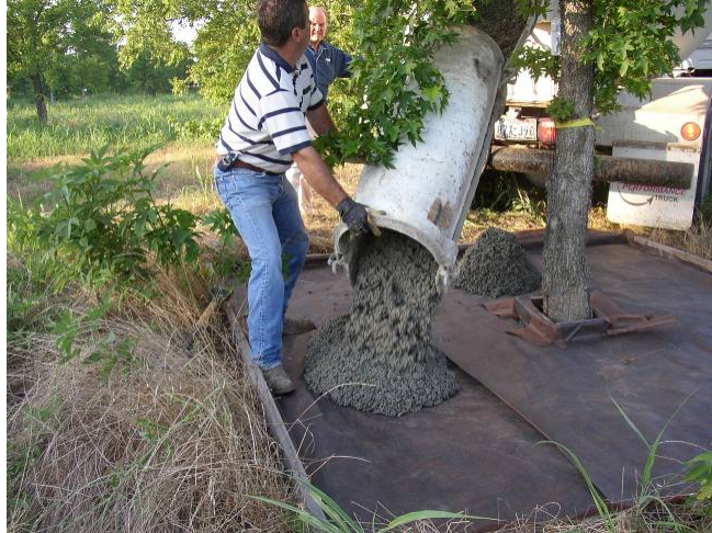
Figure 3. Installation of pervious concrete around trees.
