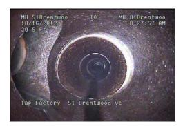
To confirm the success of the drilling operation, MSI's sewer lateral inspection units inspect the sewer mains and laterals providing video to verify the condition of the pipe after construction is complete. The inspection of the sewer main and the lateral connections is conducted from the manhole causing no more inconvenience to area residents than a standard video inspection.
