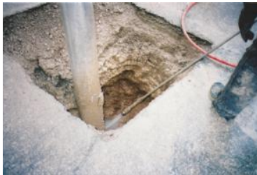
Asphalt covering problem area cut open.
