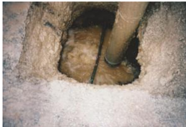
Water from broken 1" water main vacuumed into truck revealing break.
