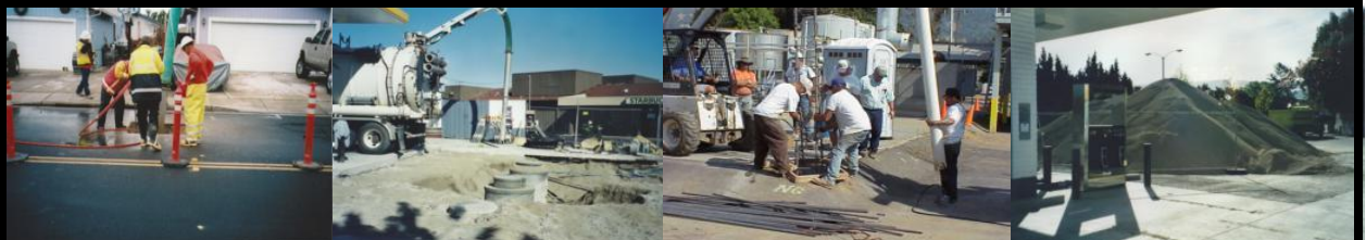
Water from broken 1" water main vacuumed into truck revealing break.
