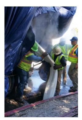
When the pipe becomes flexible but still compressed in its folded form, it is drawn through the host pipe. When the pull is complete, plugs are installed at both ends after the tow gear is removed.
