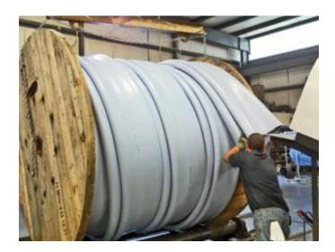
The liner arrives from the factory on spools in a rigid state, condensed and folded into an "H" shape creating a smaller profile for the pulling process. Tow gear is affixed to the liner and the steaming process begins.
