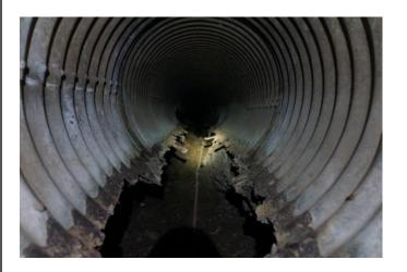
The host pipe is cleaned thoroughly, removing loose debris and roots. Conditions which would hamper the liner from being pulled through the host pipe are identified and corrected.
