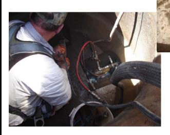
A series of solutions are injected through the hole, expanding to form a waterproof barrier and eliminate leakage.
