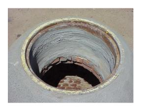
A hybrid cementitious mixture is applied to faults in the manhole to effectively plug gaps in risers and leakage from faulty seals and holes. The mixture can either be sprayed onto the manhole surface or hand applied by trowel. The mortar can be applied up to two inches thick and can be used as a stand-alone repair or to restore the manhole surface in preparation for epoxy coating.
