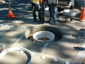
After the defective manhole has been cut away, a new chimney is sealed to the cone. The chimney is cut to allow the frame to sit flush with the surface and a quick drying concrete solution creates a tight seal collar.
