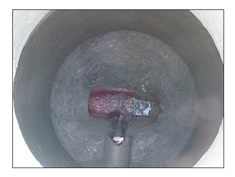
A concrete mixture is applied through a spray nozzle to coat the interior of the manhole from frame to trough creating a seamless seal.
