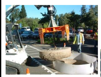
This procedure restores the manhole to the correct surface plane. In addition, defects and infiltration due to faulty risers, chimney and frame are eliminated.
