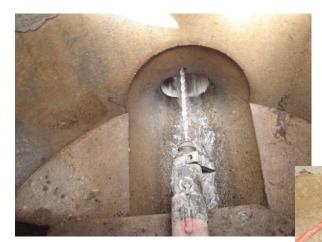
A hole is drilled to allow access to the area behind the location where leakage is a problem.
